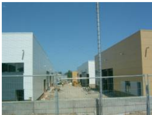
Light industrial buildings, Bray
